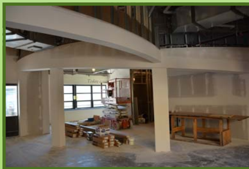
January 2016: Renovation is on schedule
