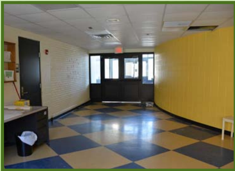
March 2015: Before the work begins
