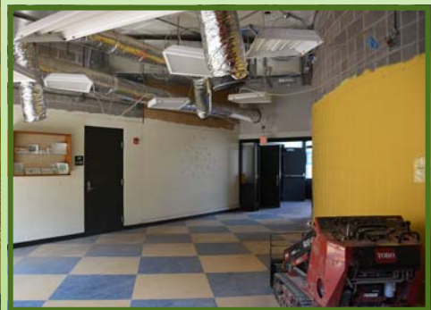
August 2015: Demolition underway
